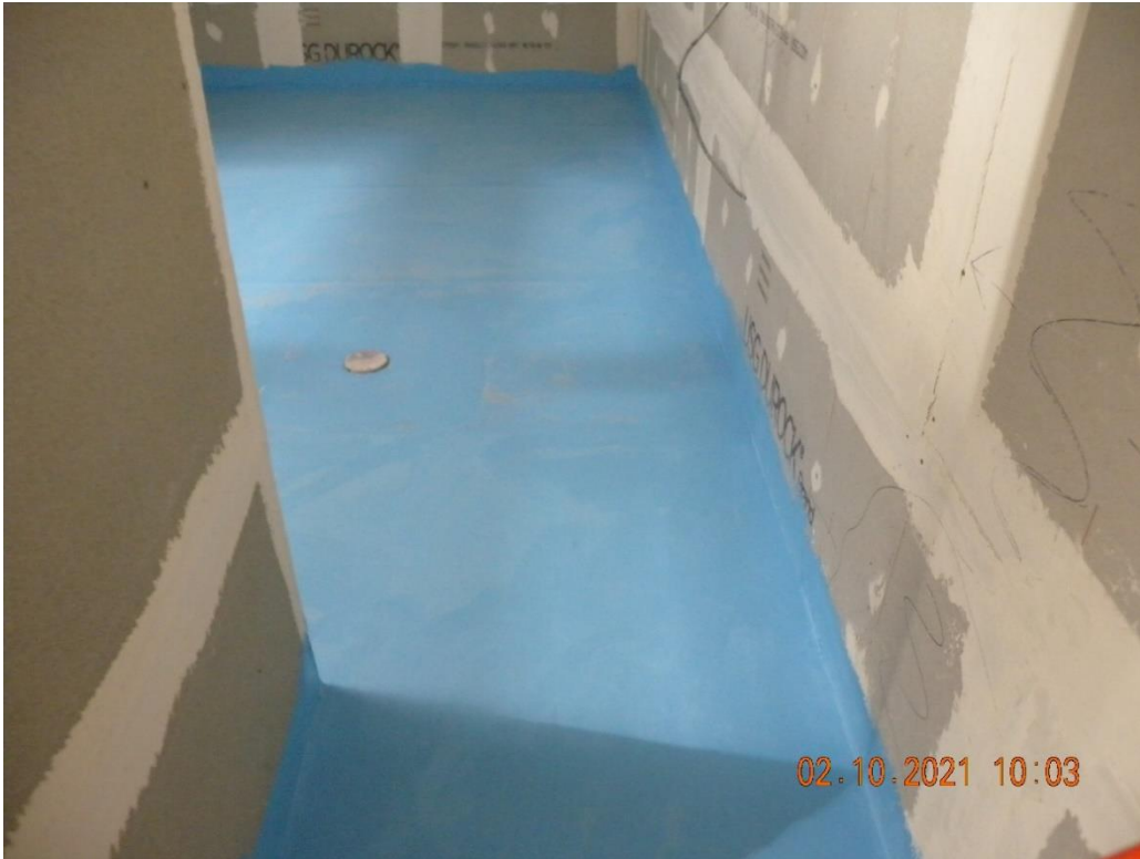
Tile worker prepared floor at bathroom third floor B Building.
