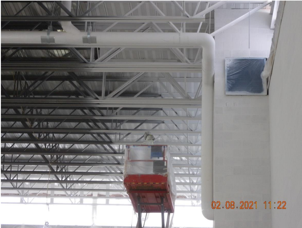
Painting Ceiling in Gym.
