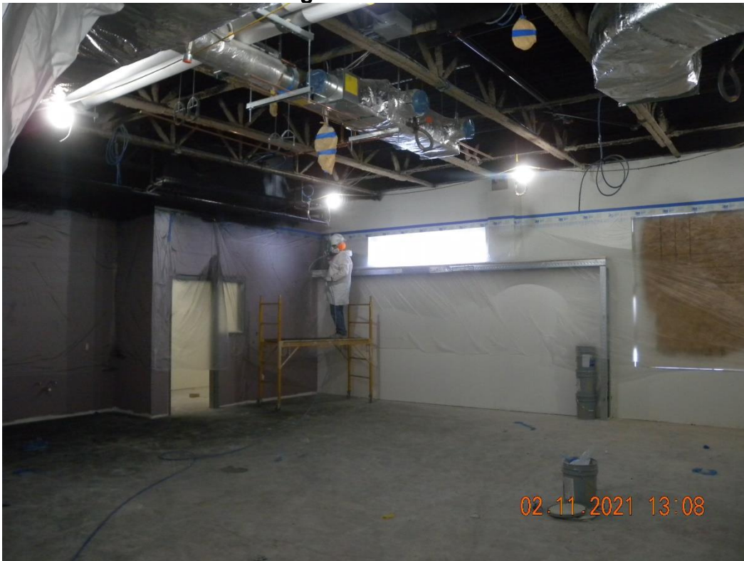
Painting walls, third floor B building.
