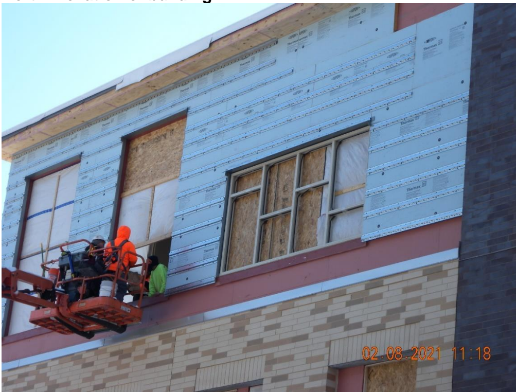
Installing metal panels at the North elevation at B
