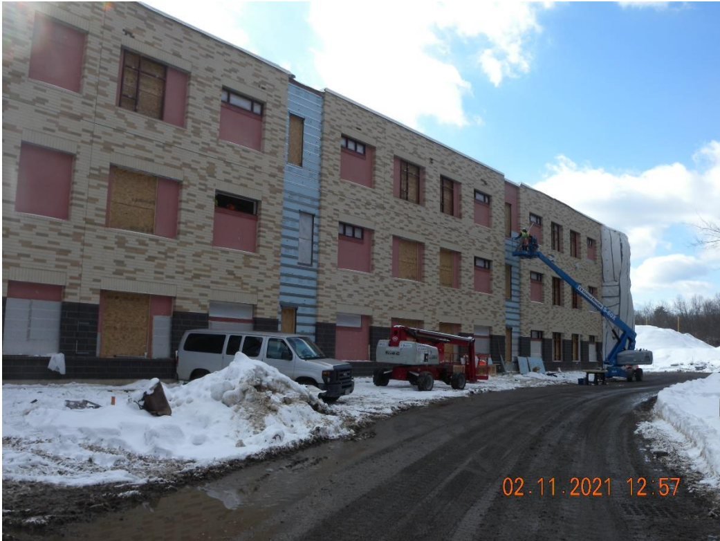
North elevation of B building.
