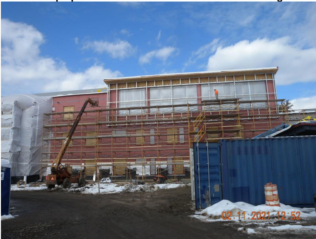
Installing staging at the remainder of South elevation of B building.
