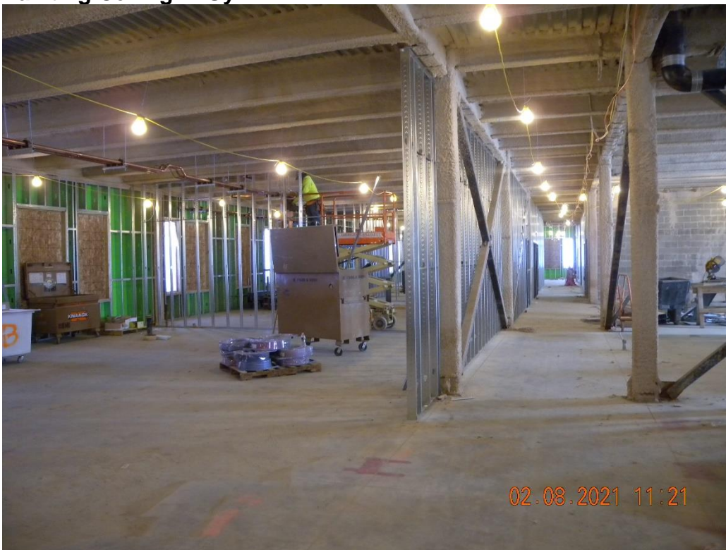
Framing first floor building D.
